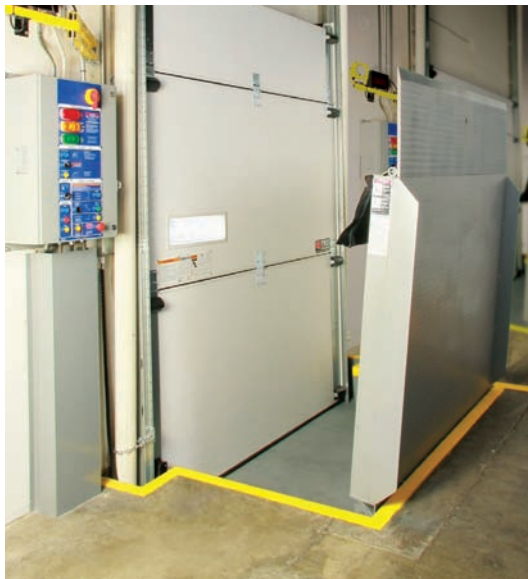
Vertical storing dock levellers with dock door.
