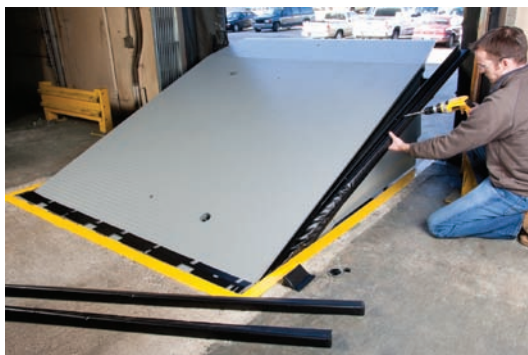
Perimeter Weather Seal – Providing a superior perimeter seal along the sides and rear of your dock leveller prevents energy loss, while blocking dirt, debris and insects.
